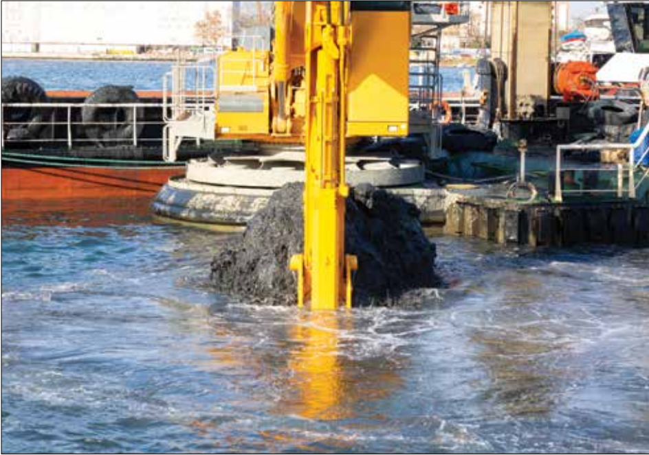
An excavator dredges a canal. (Credit: istockphoto.com/batuhan toker)
