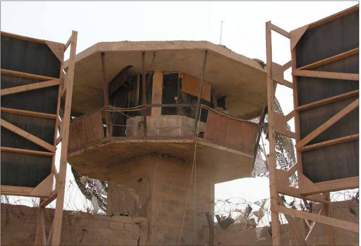
A watch tower at the Abu Ghraib Prison in 2006. (Credit: Lt. Sean Riordan)
